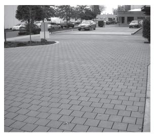
With its unique, patented interlocking spacer lugs, Eco-Priora provides secure structural performance for permeable interlocking concrete pavements (PICP's). It works well under vehicular traffic, especially when compared to other "non-interlocking" permeable pavers.
